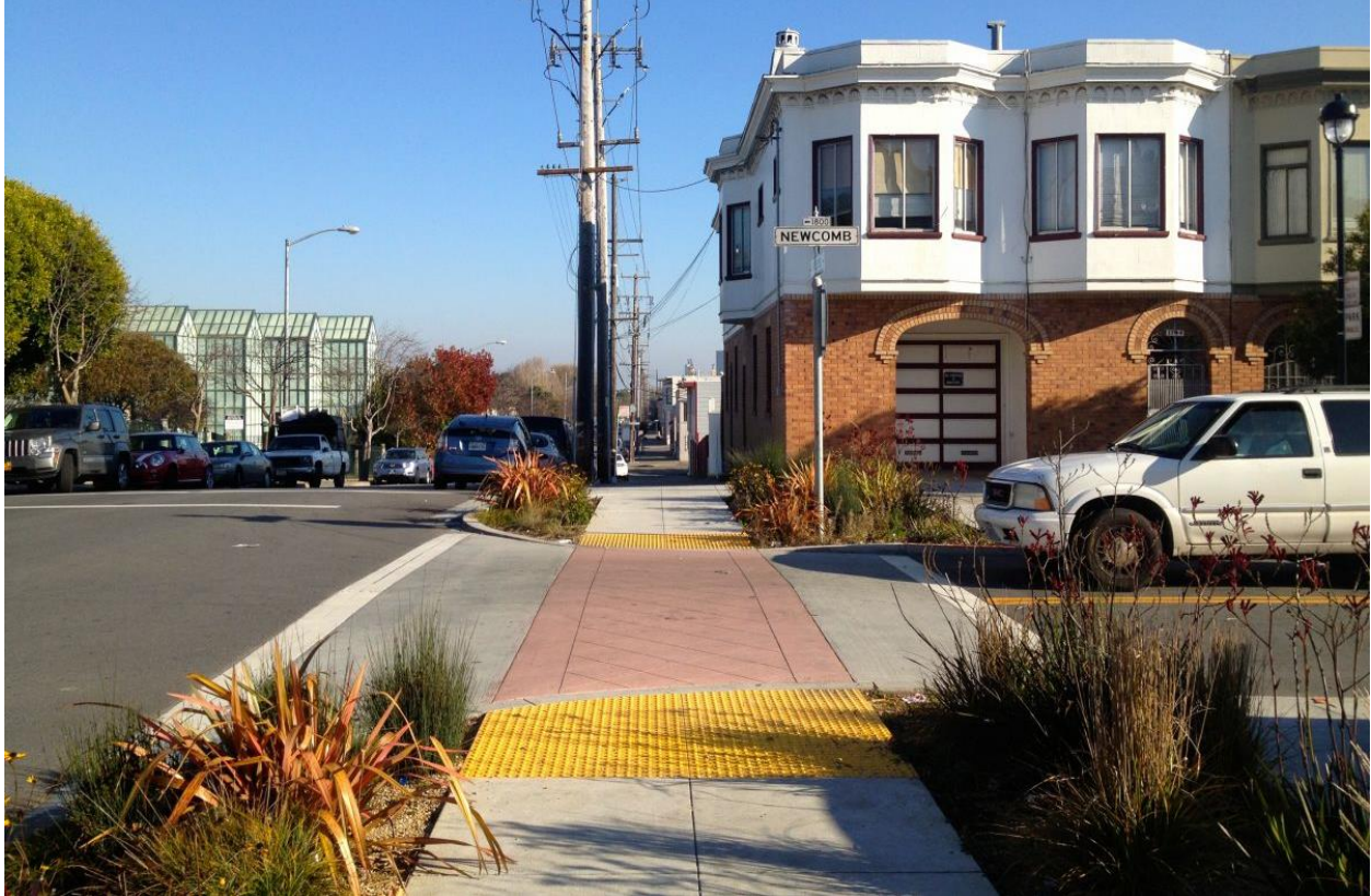
Figure 3-25. Stop-controlled intersection with dual-ramp, raised crossing, and stormwater curb extension in San Francisco. (Credit: EOA)
