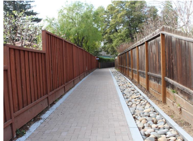
Figure 6-7. A paseo with permeable pavers and an infiltration trench connects Southgate Neighborhood to El Camino Real. (Credit: EOA)
