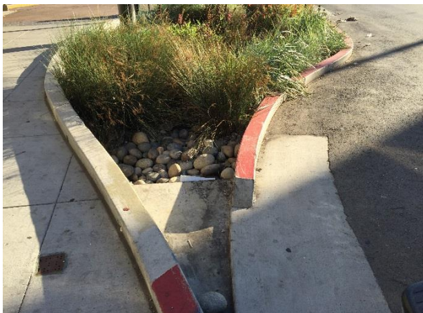
Figure 2-26. Effective curb radius for a street sweeper in San Francisco. (Credit: EOA)
