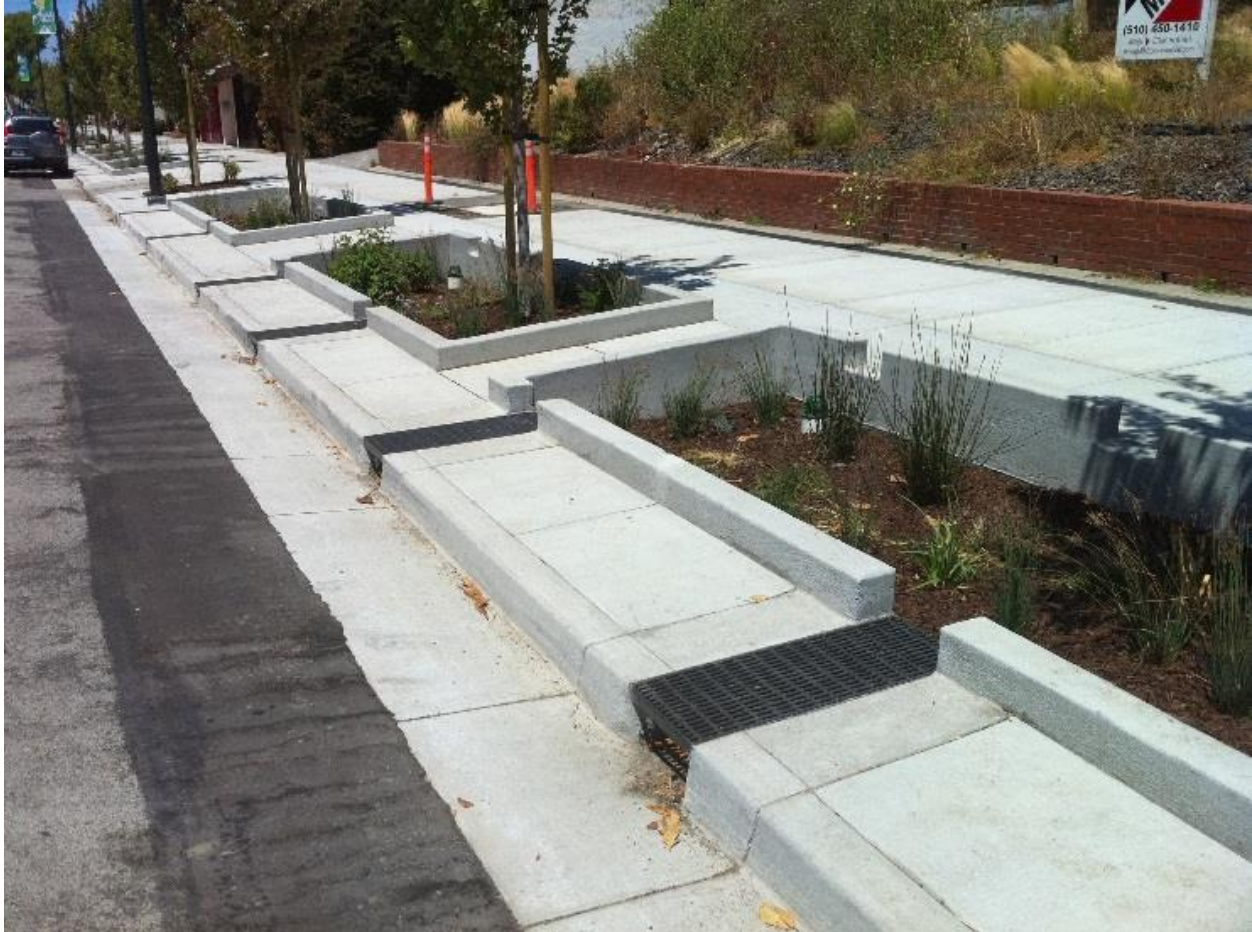
Figure 3-58. Stormwater planter with off-line flow design reducing mulch problems in El Cerrito. (Credit: EOA)
