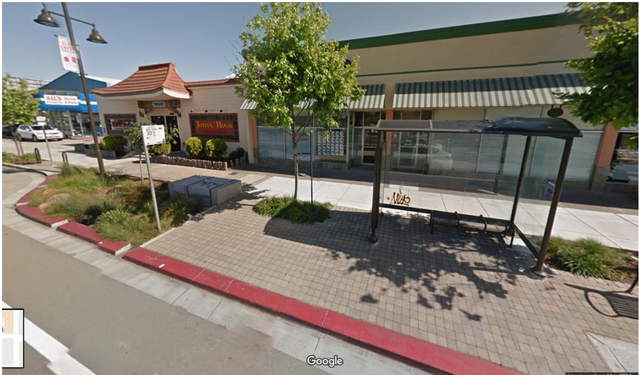
Figure 3-28. Midblock transit stop with pervious pavement and stormwater curb extension in Castro Valley. (Credit: Google Street View)
