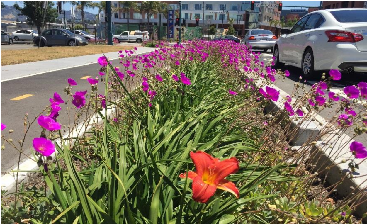
Figure 3-17. Stormwater planter between cycletrack and roadway in Emeryville. (Credit: EOA)
