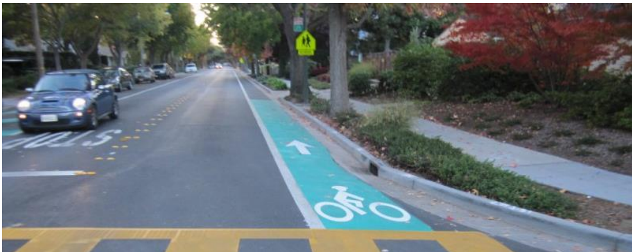
Figure 2-10. Class II bicycle lane with green pavement in Palo Alto. (Credit: Palo Alto Patch)
