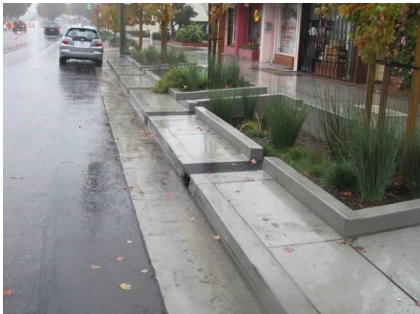
Figure 4-2: Off-line system in El Cerrito where low flow is diverted to the sidewalk planter and high flows continue down the gutter.
