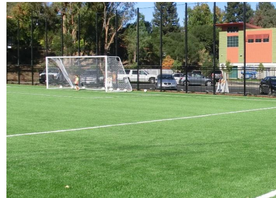
Figure 6-23. Synthetic turf design allows infiltration on site. (Credit: EOA)
