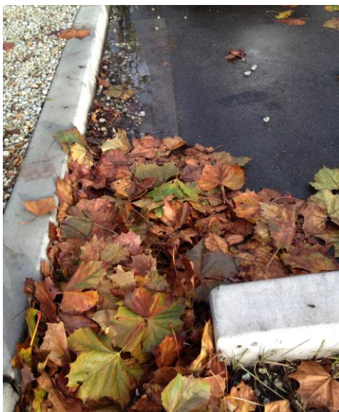
Figure 3-43. London plane tree leaves blocking a stormwater curb extension inlet in Emeryville. (Credit: EOA)
