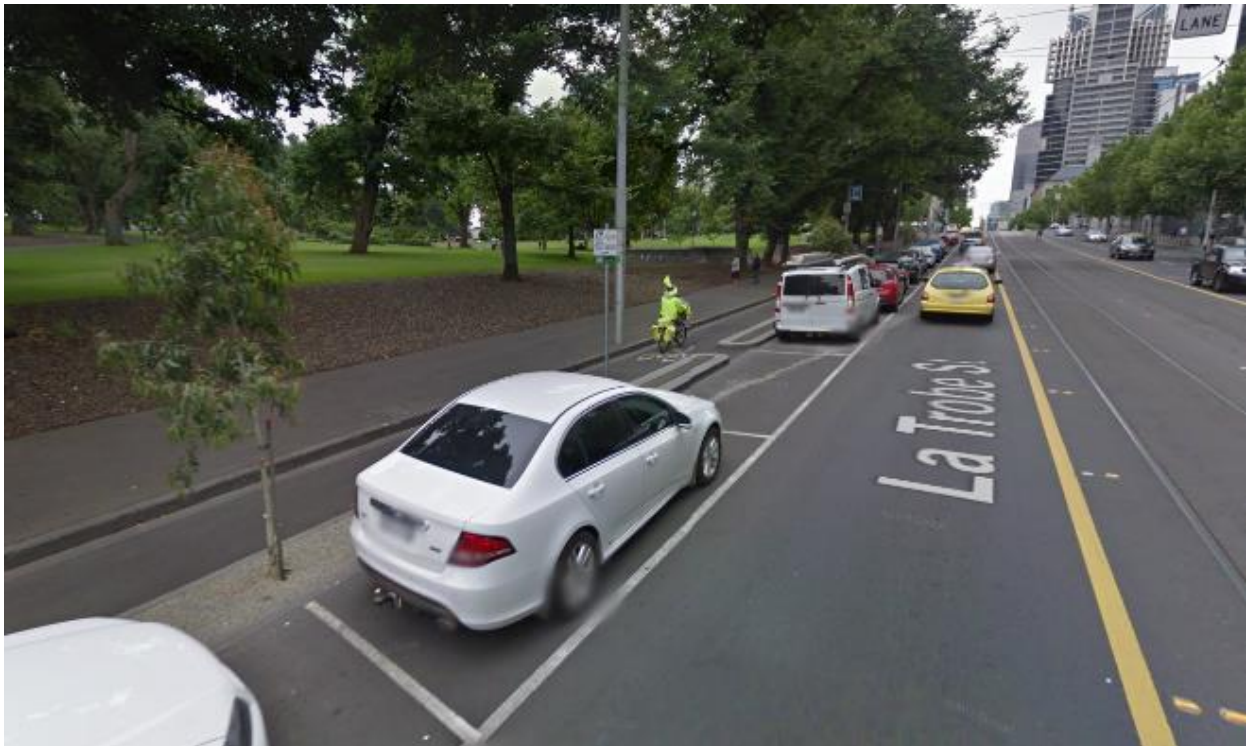
Figure 2-15. After: cycletrack with raised median, street trees & parked cars. (Credit: Google Street View)
