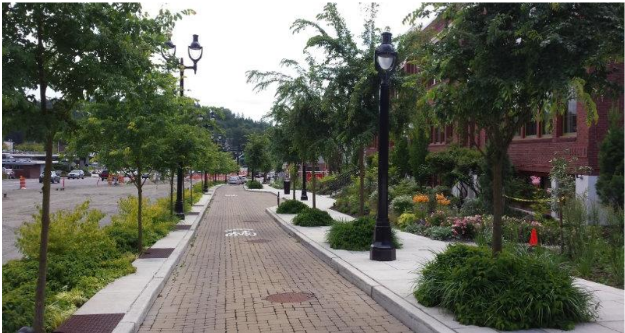
Figure 3-12. One-way, class III bikeway with pervious pavement and Silva Cells for street tree planting in Bothell, WA. (Courtesy of DeepRoot GSI, LLC)
