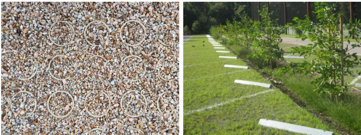
Figure 2-37. Grid paving in a parking lot in Napa (Left) and in a parking lot in Cupertino (Right). (Credit: EOA and Cupertino)
