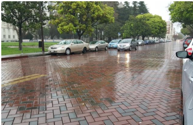
Figure 6-13. Pervious pavement installed in Allston Way, Berkeley. (Credit: URS)
