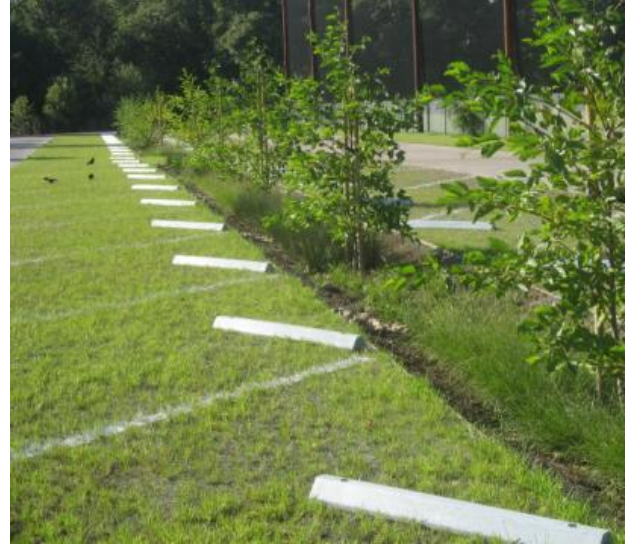
Figure 6-27. The plantable geocells are backfilled with special soil. During heavy rains, excess water flows to bioretention areas in center. (Credit: Cupertino)
