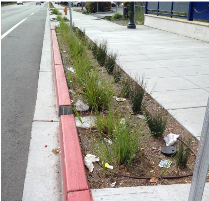
Figure 3-64. Litter needing manual collection in a stormwater planter in the City of San Mateo. (Credit EOA)
