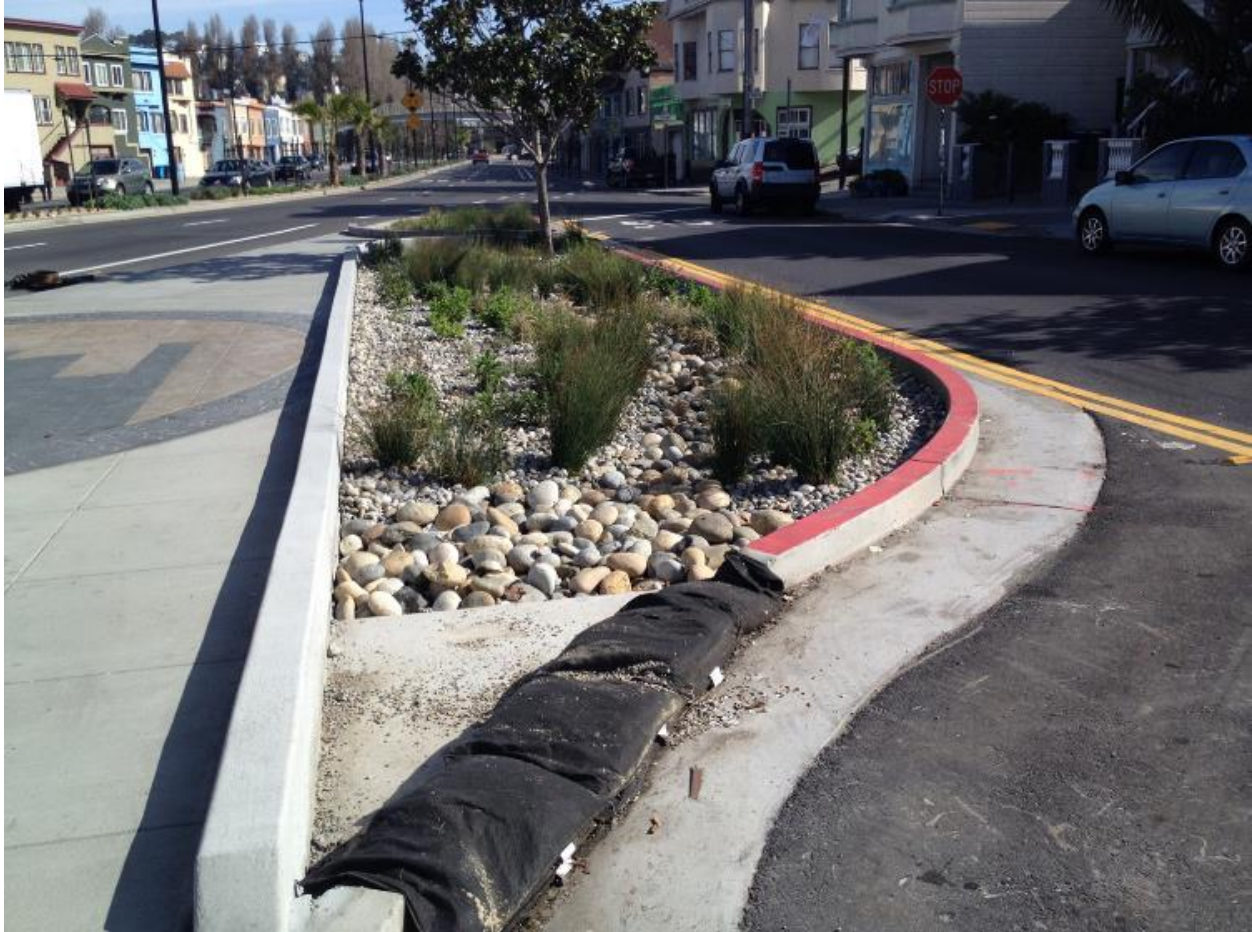
Figure 3-63. Gravel bags protect a stormwater curb extension during plant establishment in San Francisco. (Credit: EOA)
