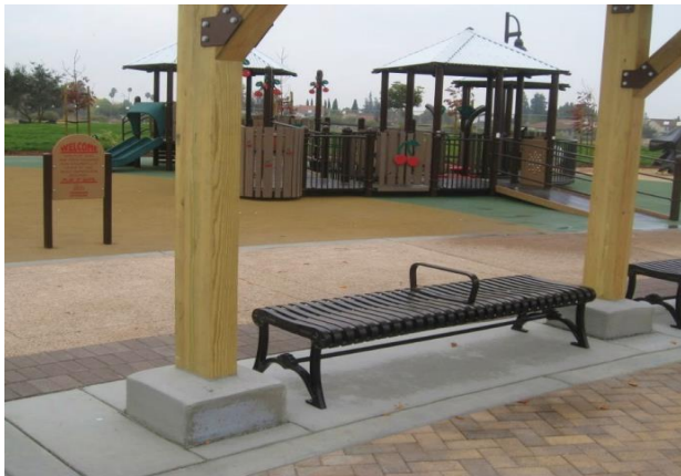
Figure 6-18. The park contains porous rubber surfacing in the play area and pervious concrete in walkways. (Credit: San Jose)
