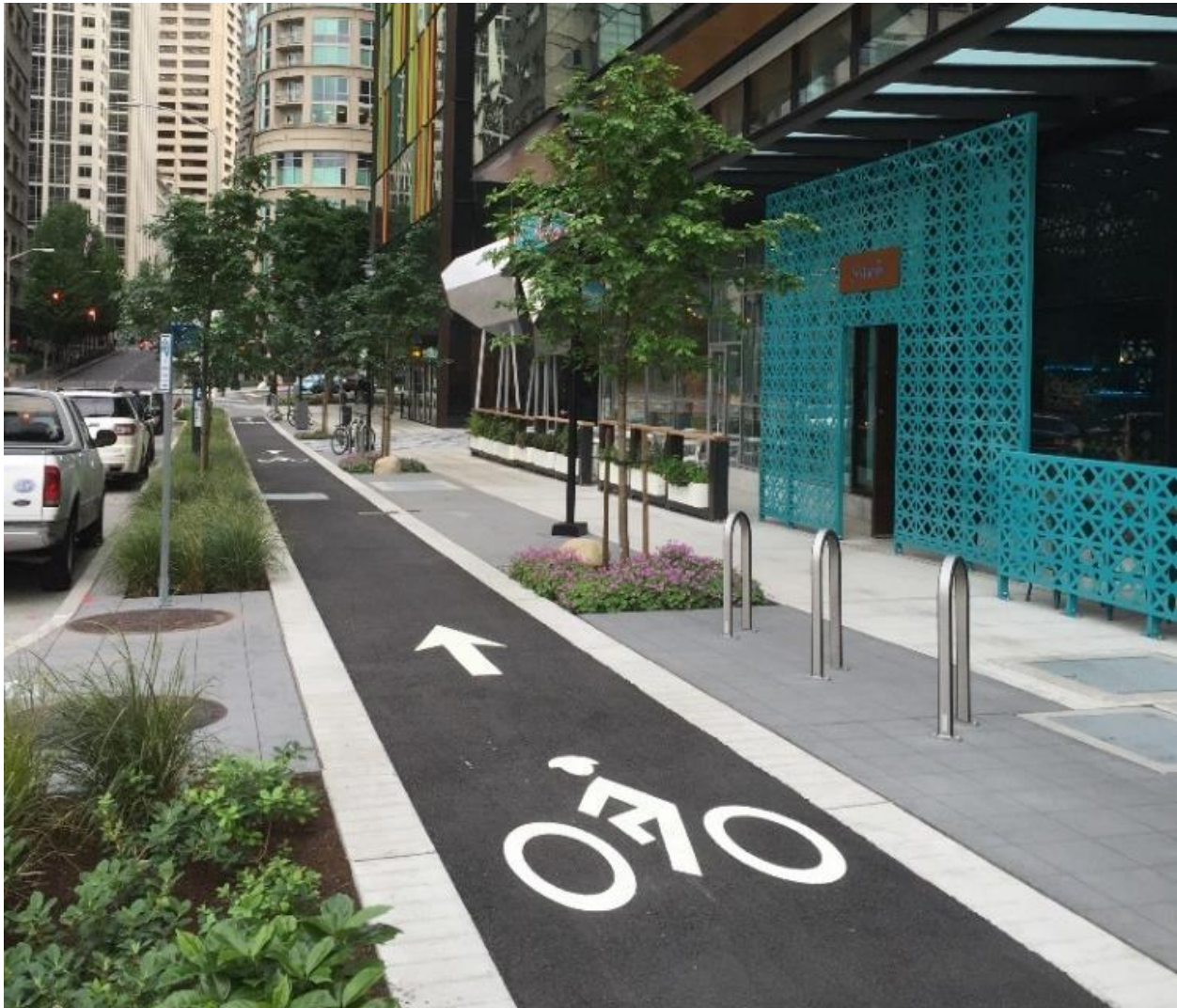
Figure 3-48. Stormwater tree well filter with suspended pavement and cycletrack in Seattle. (Courtesy of DeepRoot GSI, LLC)
