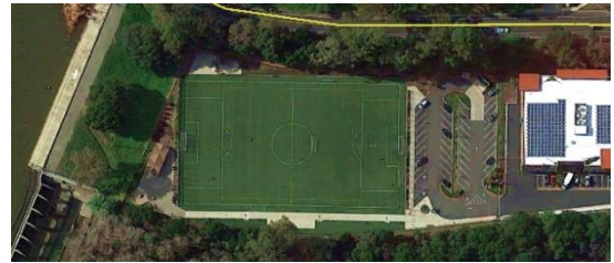
Figure 6-22. Park site before and after project. (Credit: Los Gatos)
