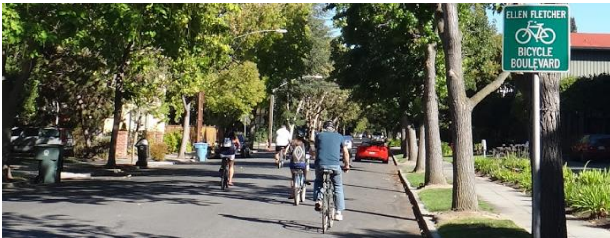
Figure 2-12. Class III bicycle boulevard in Palo Alto. (Credit: https://bikeaway.tumblr.com/post/30365628672/bay-area-aqain-tunitas-creek-old-la-honda-and )
