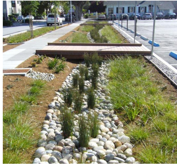
Figure 6-17. Bioretention area between parking lot and sidewalk features native California plants. (Credit: Burlingame)
