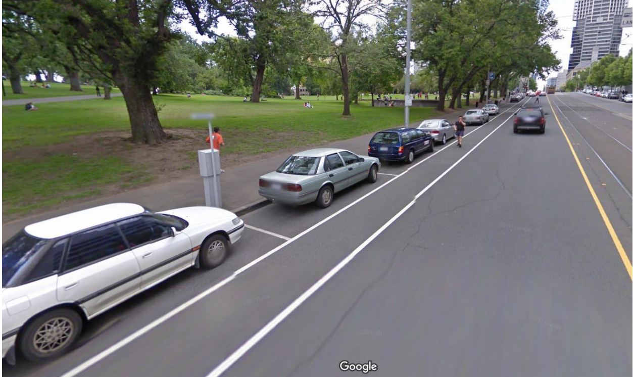
Figure 2-14. Before: standard unprotected bicycle lane in Melbourne, Australia (Credit: Google Street View)
