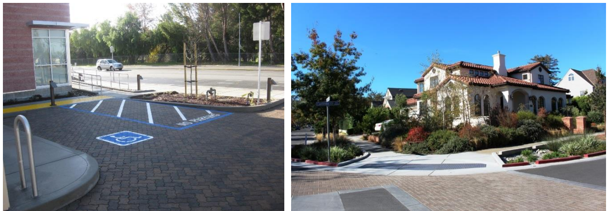
Figure 2-36. Permeable pavers at Fire Station 21 in San Jose (left) and in a crosswalk in Palo Alto (right). (Courtesy of Pacific Interlock Pavingstone & the City of Palo Alto)
