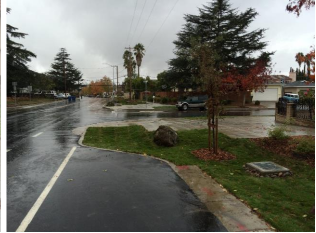
Figure 6-3. Stormwater curb extension at an improved intersection. (Credit: EOA)
