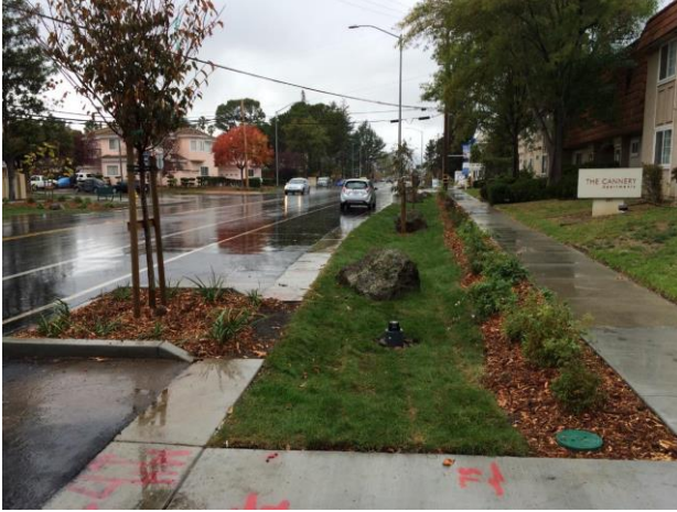
Figure 6-2. Stormwater planter along Hacienda Avenue with connection to a tree well filter. (Credit: EOA)
