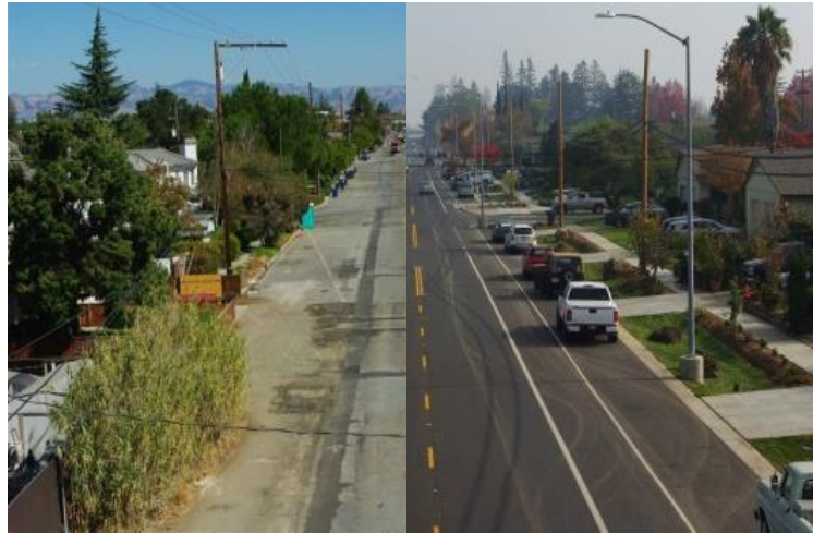
Figure 6-1. Hacienda Avenue before and after improvement project. (Credit: City of Campbell)
