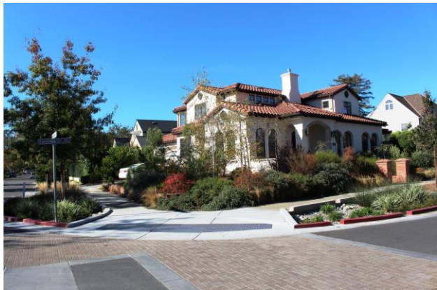
Figure 6-4. Southgate Neighborhood project bioretention areas and pervious pavement on crosswalks. (Credit: City of Palo Alto)
