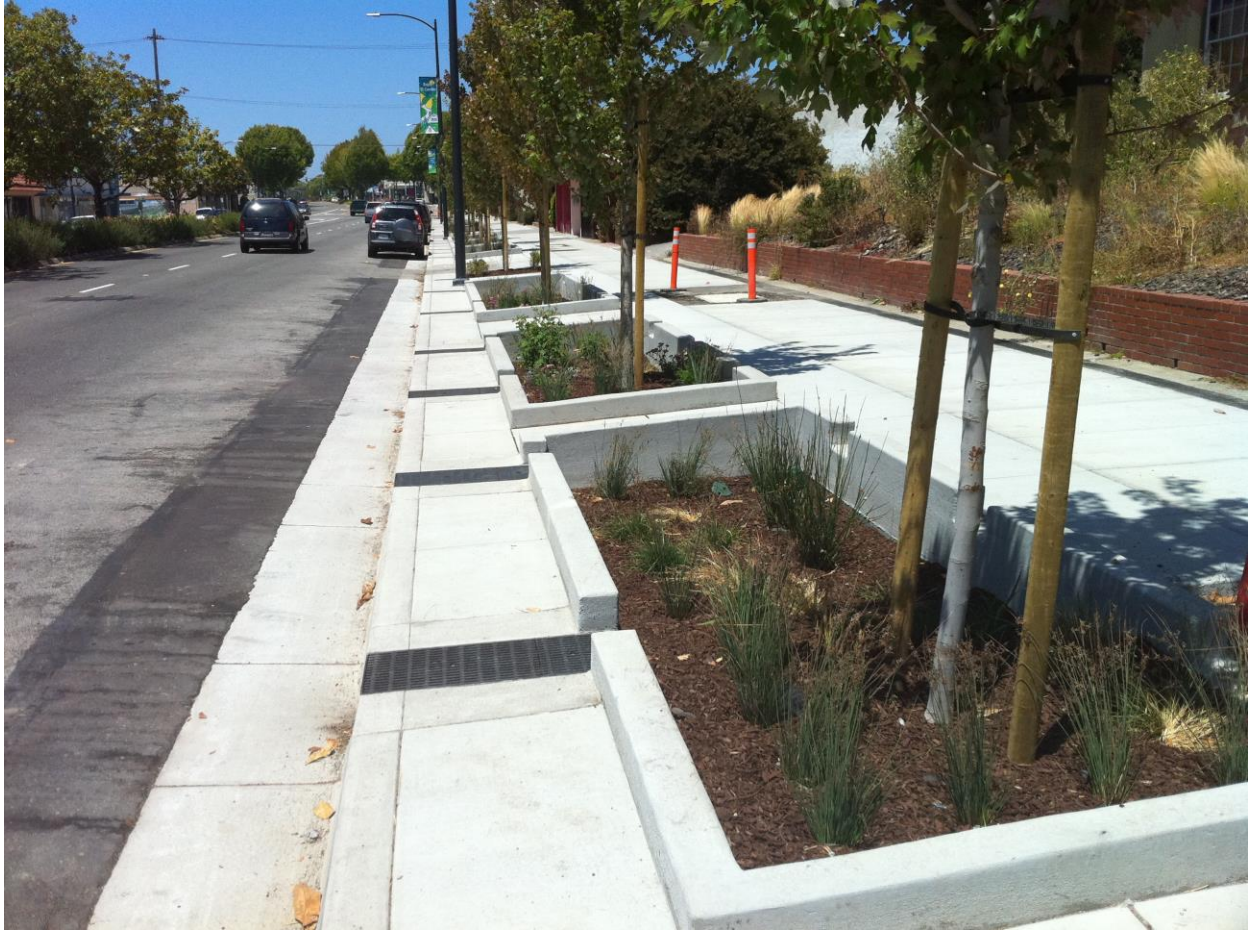
Figure 2-19. Stormwater planter with vertical sides, step-out zone and on-street parking in El Cerrito. (Credit: EOA)
