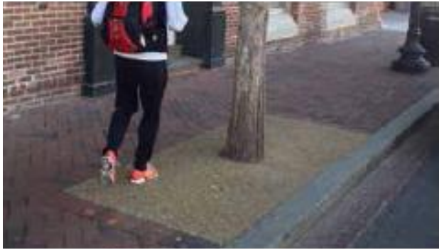
Figure 2-34. Porous rubber example. (Courtesy of DDOT)
