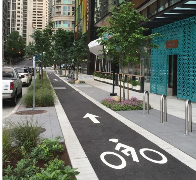
Figure 3-13. One-way, raised cycletrack with a suspended pavement system in Seattle (stormwater tree well filter with cycletrack). (Courtesy of DeepRoot GSI, LLC)
