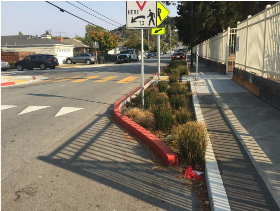
Figure 3-35. Laurel Elementary School, City of San Mateo, Safe Routes to School project includes stormwater curb extension. (Credit: EOA)
