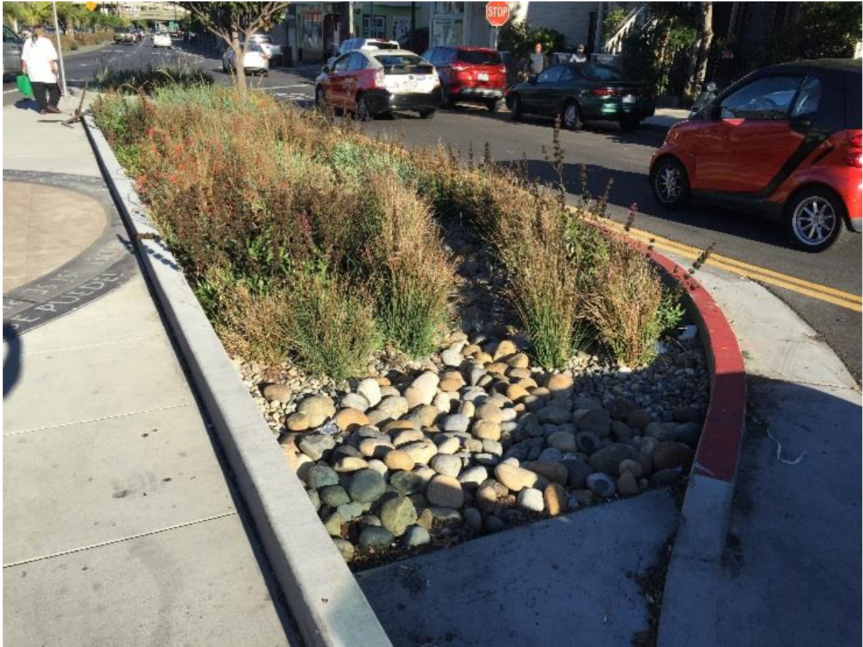
Figure 3-59. Stormwater curb extension with in-line flow design using rock cobbles & rock mulch in San Francisco. (Credit: EOA)
