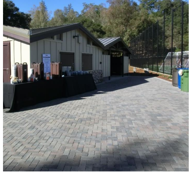
Figure 6-25. Permeable pavers are used in park plazas, walkways, and picnic areas. (Credit: EOA)
