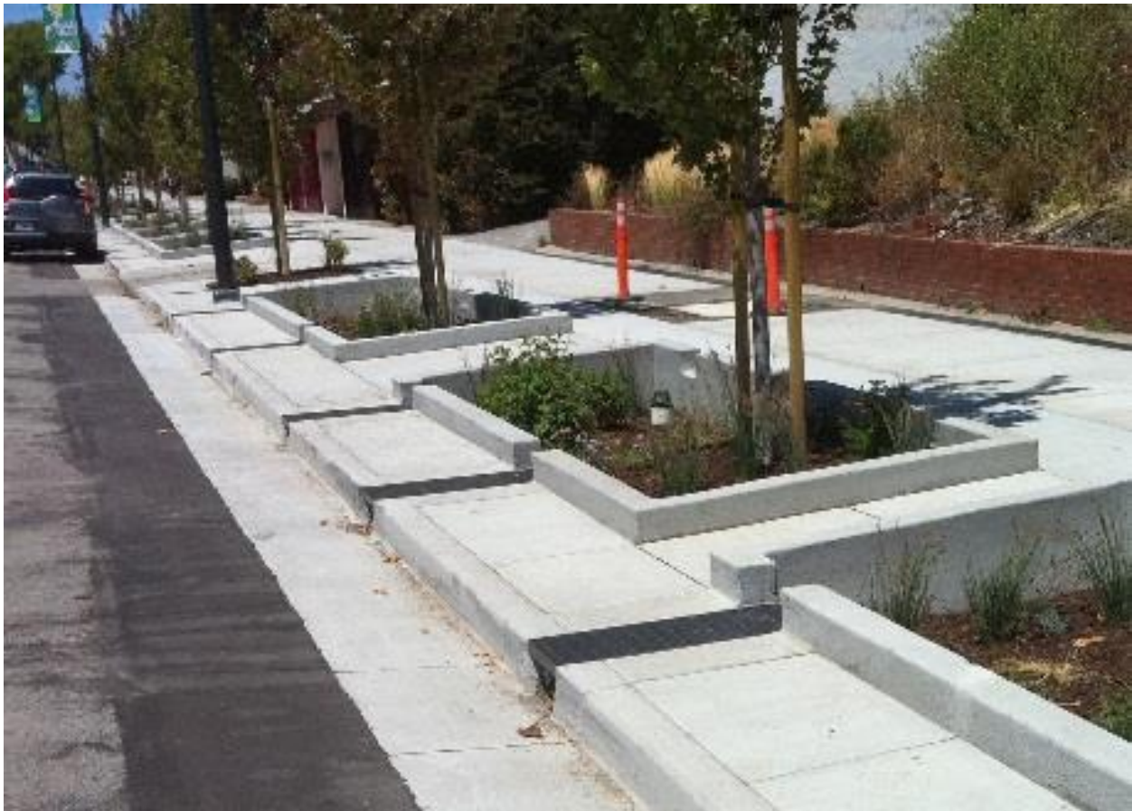
Figure 6-12. Completed stormwater planters along San Pablo Ave. (Credit: EOA)
