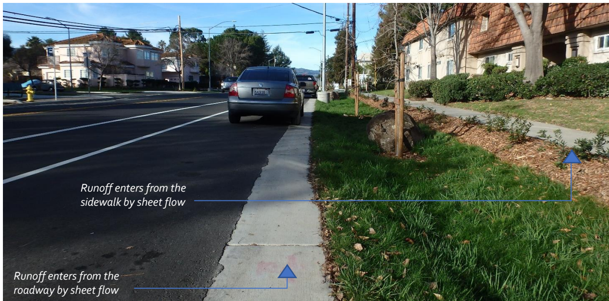
Figure 2-16. Stormwater planter on Hacienda Avenue in Campbell. (Credit: EOA)
