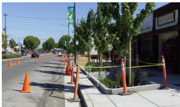
Figure 6-11. Biotreatment areas after planting at Eureka site. (Credit: El Cerrito)
