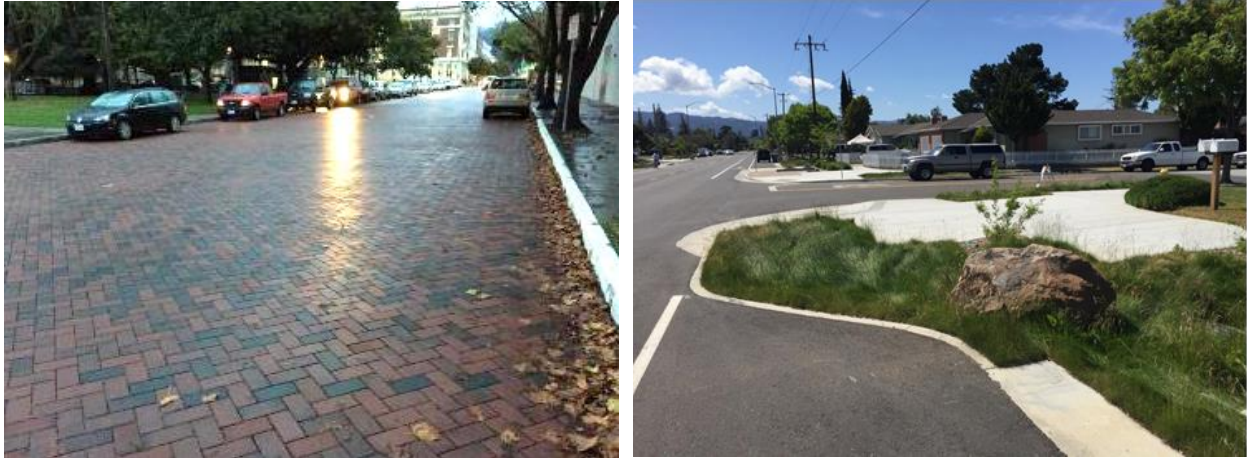
Figure 3-20. Pervious pavement, Allston Way, City of Berkeley (left); stormwater curb extension, Hacienda Avenue, City of Campbell (right). (Credit: EOA)
