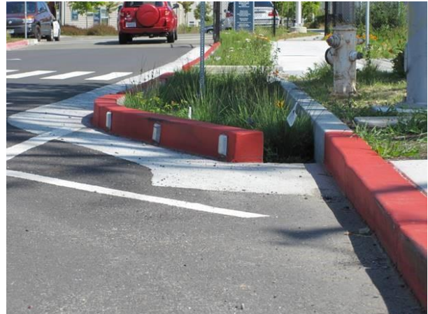
Figure 4-1: In-line system in Berkeley/Albany where low and high flows enter the system and overflows exit through a drain within the system.
