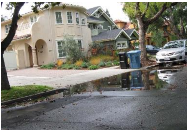
Figure 6-5. Localized ponding before green stormwater infrastructure upgrades in the Southgate Neighborhood. (Credit: Palo Alto)
