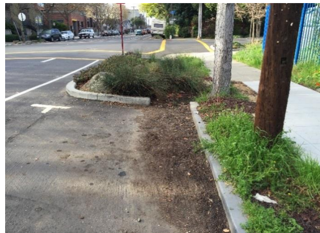
Figure 2-27. Ineffective curb radius for street sweeper in Emeryville. (Credit: EOA)
