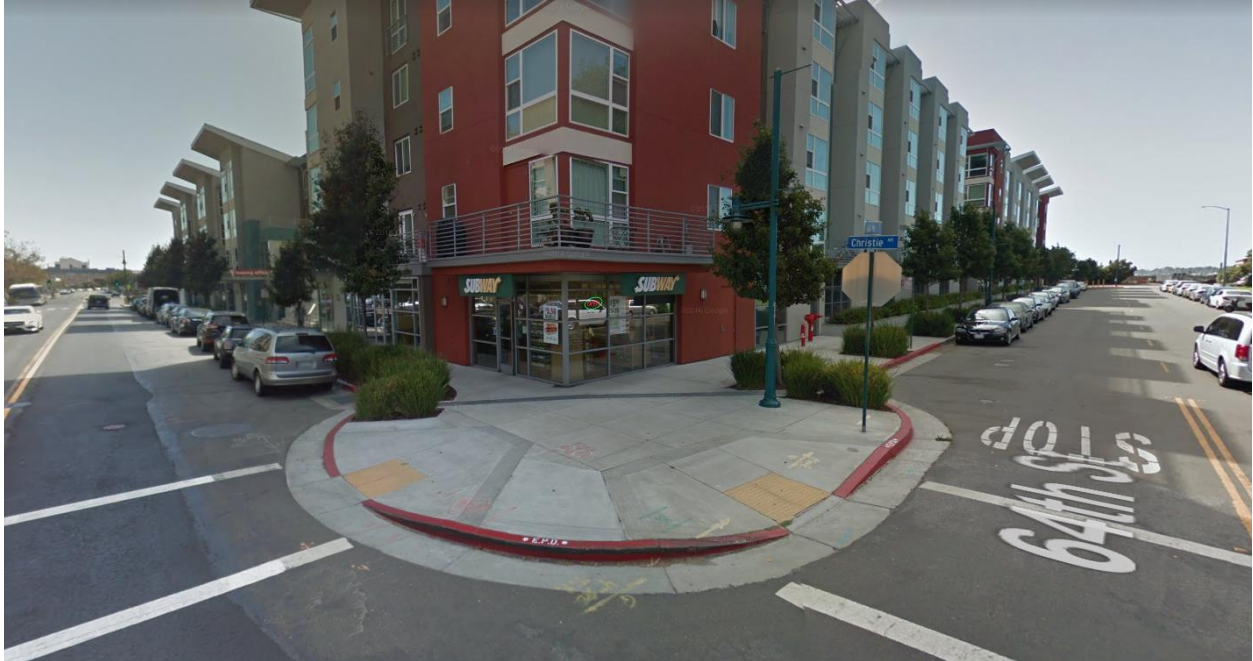
Figure 3-27. Stop-controlled intersection with dual ramp, raised curb, street-level crossing, and standard curb extension with trench drain in Emeryville. (Credit: Google maps)
