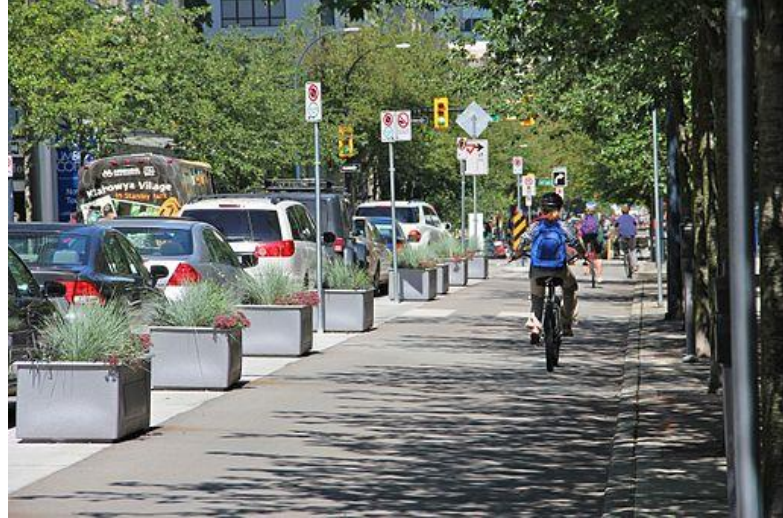
Figure 3-15. Moveable raised planter boxes can be used to test a new cycletrack installation such as this one in Vancouver on Hornby Lane. (Credit: https://commons.wikimedia.org )
