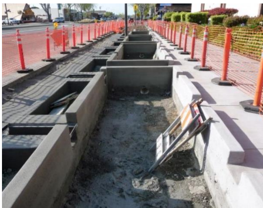
Figure 6-10. Cells in construction at Madison site. (Credit: El Cerrito)
