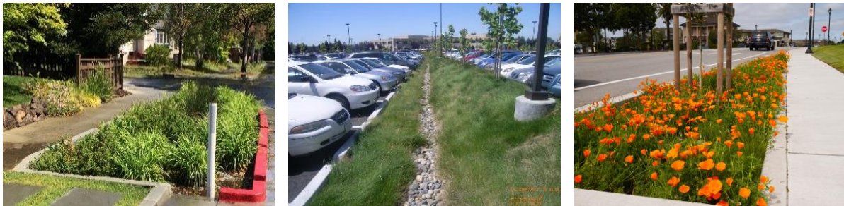
Figure 3-36. Examples of GSI landscape designs. (Credit: Cities of Palo Alto and San Jose and Urban Rain Design)
