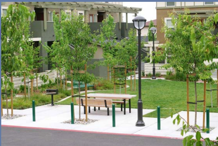
Sara Conner Court, Affordable Housing, Hayward
