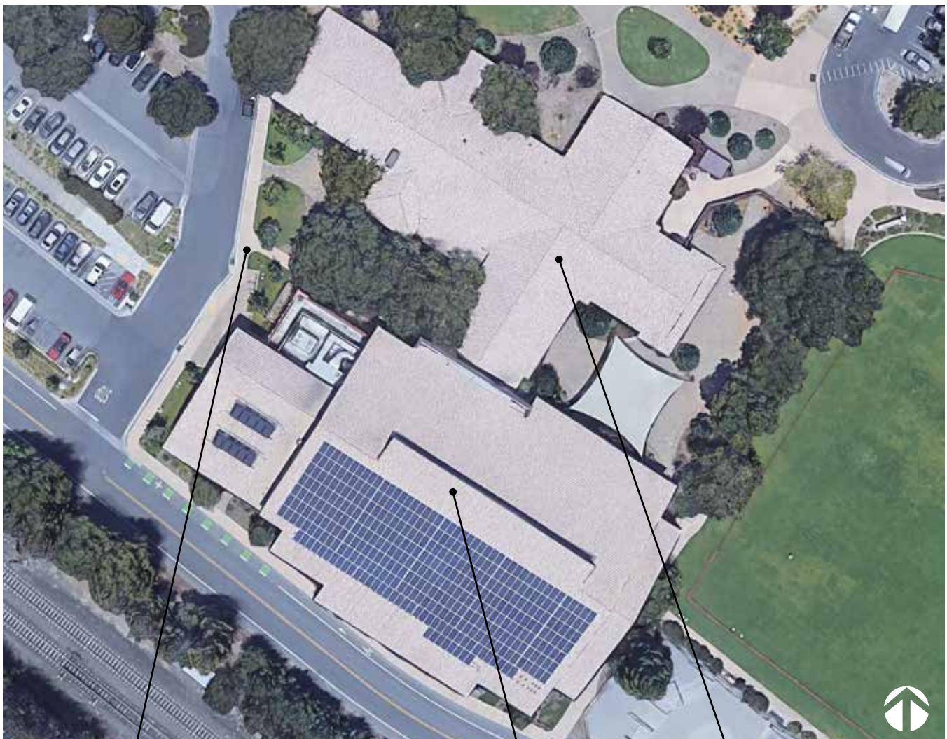
Potential future addition connecting the two buildings and adding a fitness center
